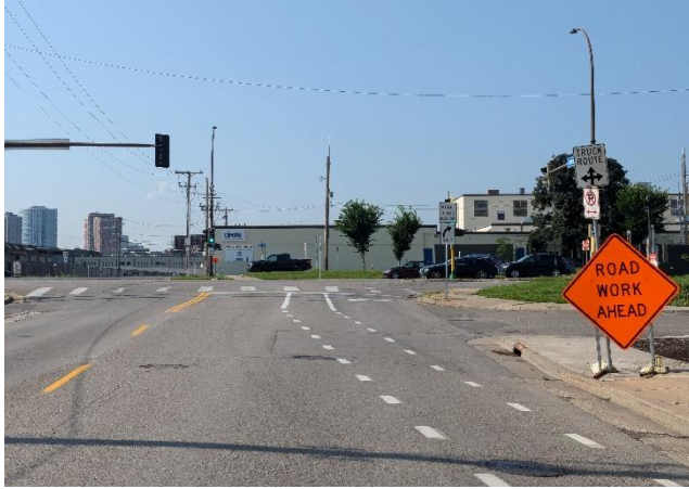
Figure 51 Missing marking and signage for through bike lane.
