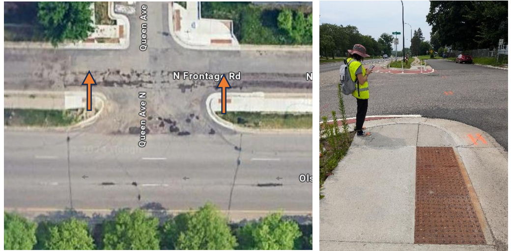
Figure 26: Curb cuts do not align for crossing Queen Avenue. Bollards also placed in the path of travel when crossing Queen Avenue. (photo on right)
