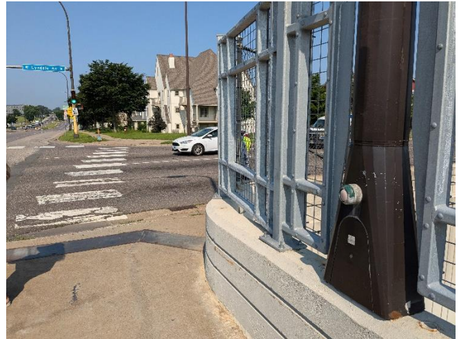
Figure 37 Pedestrian signal button setback from crossing with missing signage.
