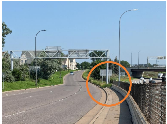
Figure 38 Sidewalk ends with no safe crossing facility.
