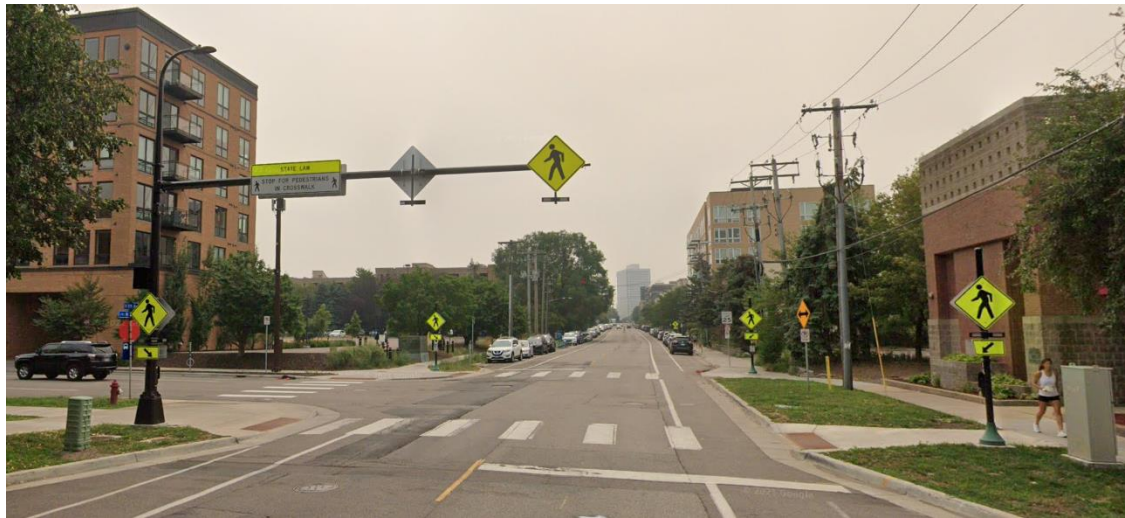
Figure 15 Example of a Rectangular Rapid Flashing Beacon (RRFB) and pedestrian crossing signage installed at 8 th Ave and 2 nd St. in Minneapolis
