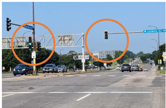
Figure 43 Overhead traffic light not visible compared to post-mounted light.
