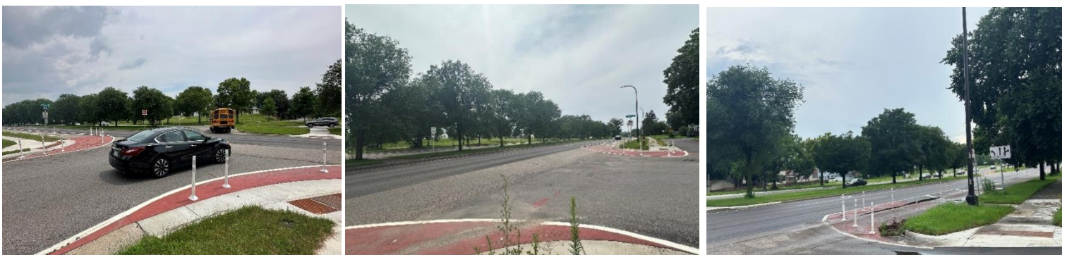
Figure 17 Wide turning radii on turns.
