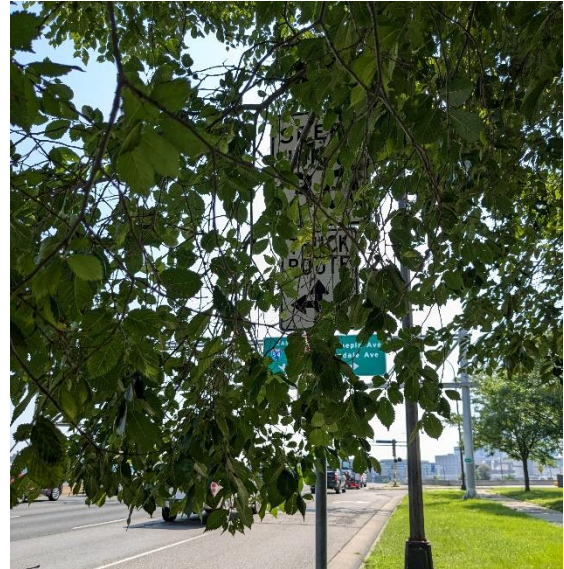
Figure 39 Obscured visibility of speed limit sign.
