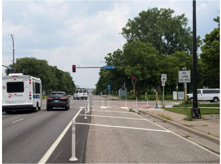
Figure 30 No turn on red sign.
